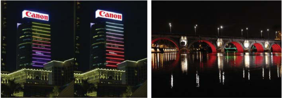
Figure 1.12. Left: LED illumination of the Canon tower in Kowloon (Hong Kong) 14 lines with 30 LEDs per line. Each chip consumes 6 W and includes six junctions (2 red, 2 green and 2 blue), for a total power of 12.5 kWh per night [LED 07]; right: arches of the Pont Neuf bridge in Toulouse have been illuminated since November 2007 with a dynamic LED lighting (total power 1 kW)
